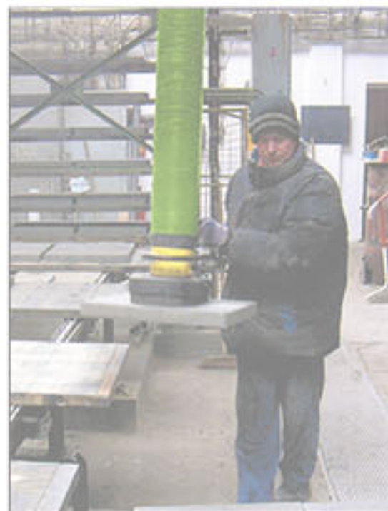
▲ 塑板搬運作業 Plastic Plank / brick
